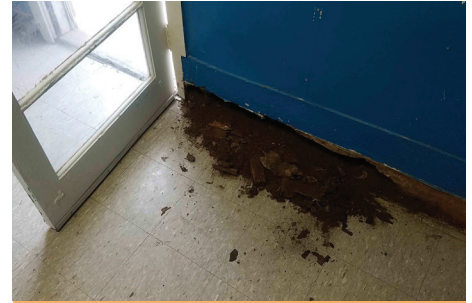
Termite Damage
